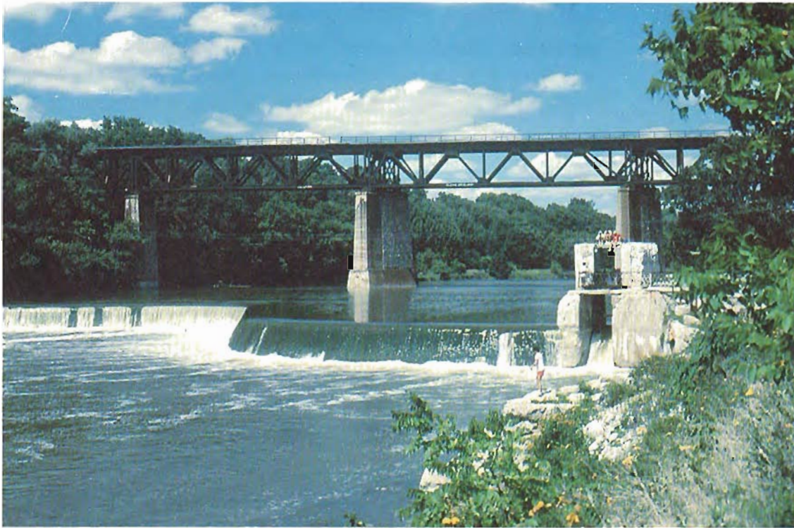
Built in the 1870s, Penman's Dam provided water power for textile mills on the Grand River in Paris.
