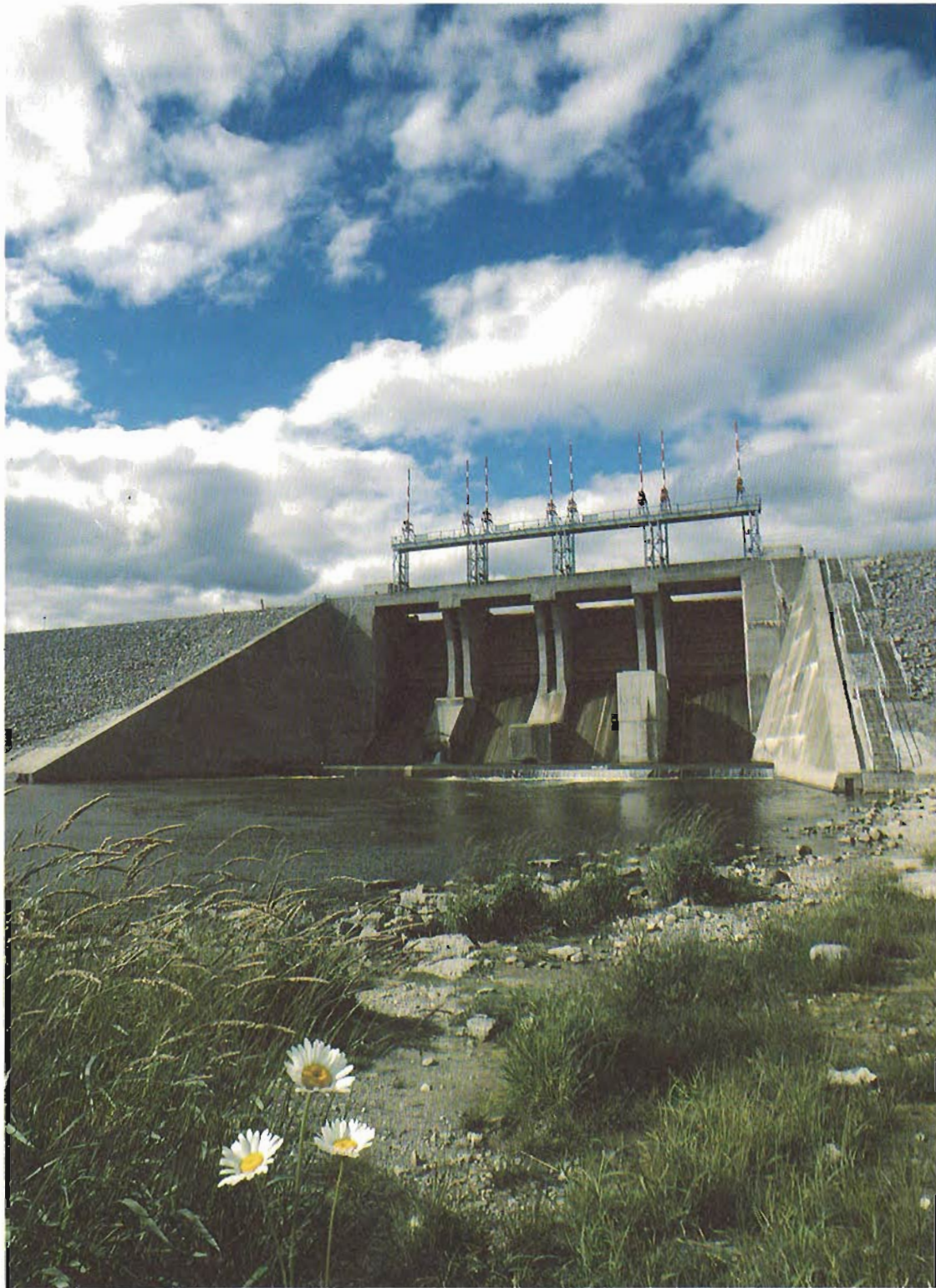
Located north of Fergus on the Grand River, the Shand Dam, built in 1942, was the first multi-purpose dam in Canada and became the model for other water control structures in Ontario and Canada. John deVisser
